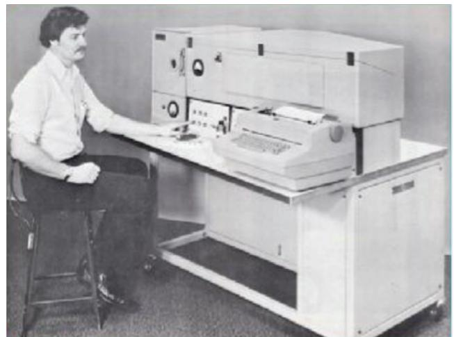
**Figure 5:** A Direct Reading Oil Analysis Spectrometer from the 1970's
